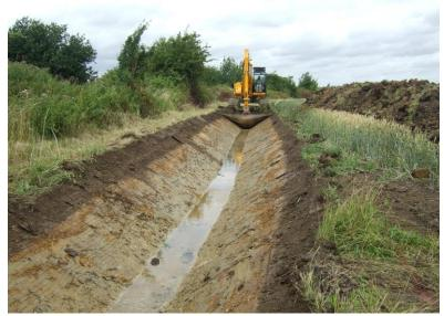
Figure 10-1: Completed action to create a new ditch near Eye Green to reduce flooding
